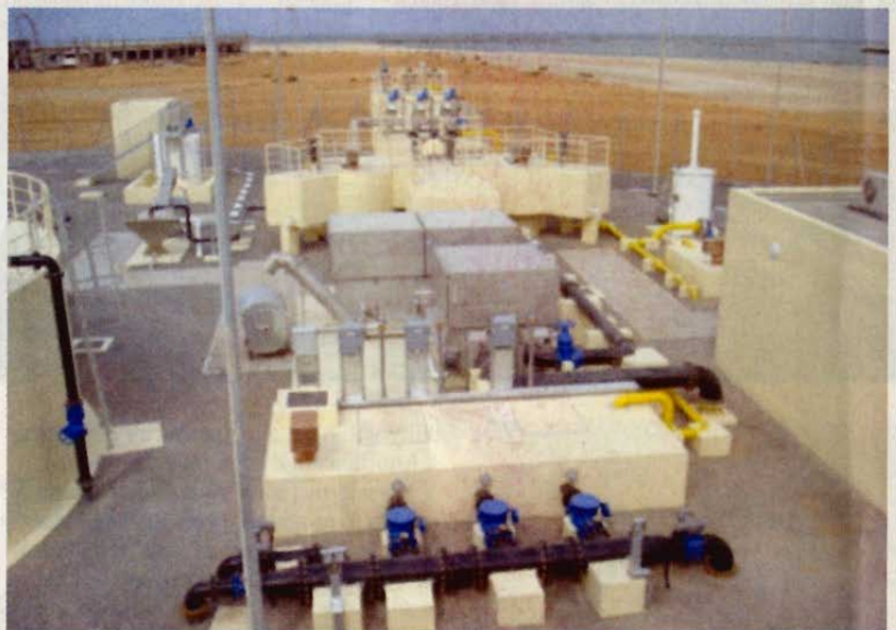
Mina Al Arab sewage treatment plant
